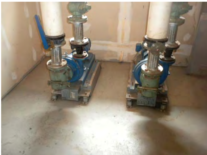
The heating water circulator pumps
