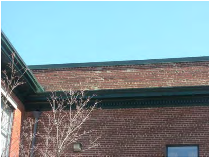
Spalling brick and mortar loss typical of the original building
