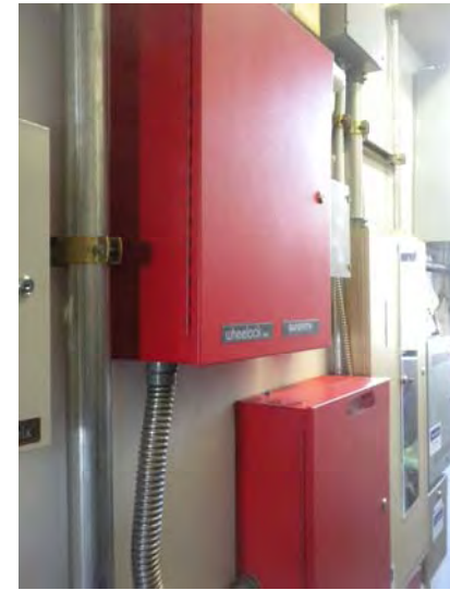
The central fire alarm control panel
