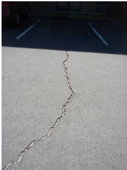
Example of cracking parking area
