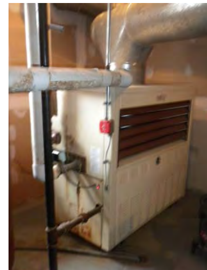
The domestic hot water boiler
