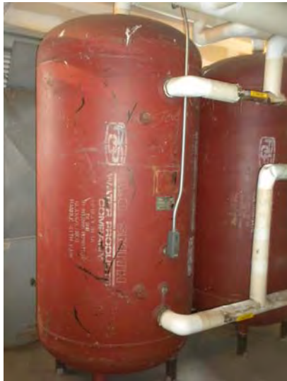
Domestic hot water storage tanks
